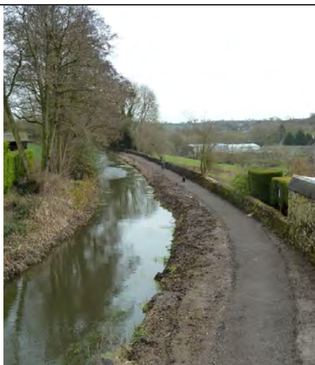
During and after dredging at Ambergate. The towpath has been fully resurfaced. Photos: Hugh Potter
