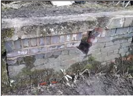
Brickwork repaired; compare this to the photograph on page 24.
