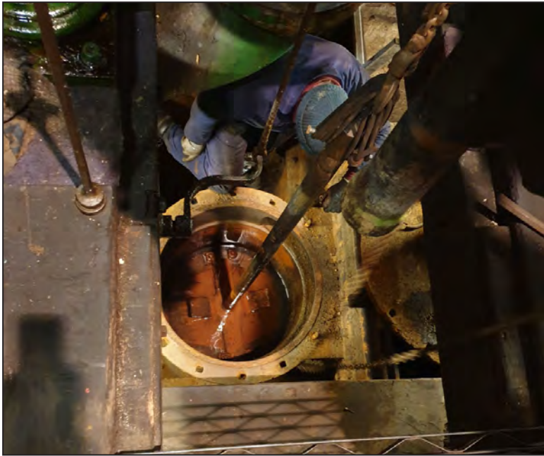
The air pump being removed. Photos: Mike Lewis
