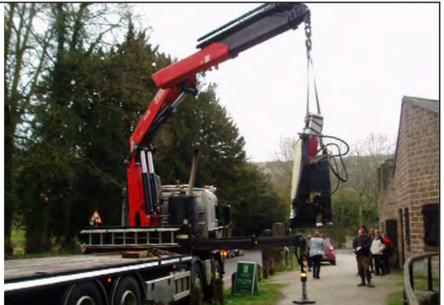
Swinging the rudder assembly onto the lorry for transport to Langley Mill workshop. Photo: John Baylis
