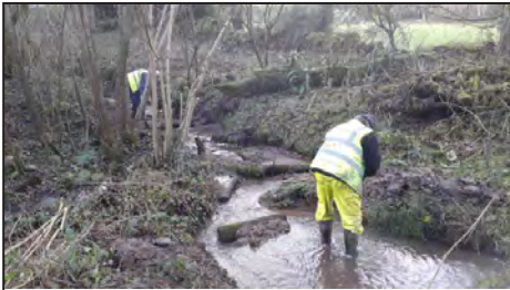
Clearing silt traps.
