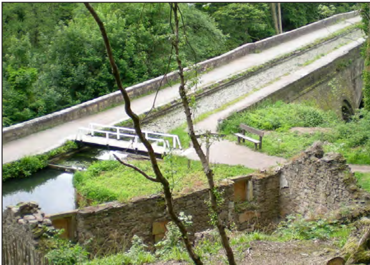
Derwent Aqueduct seen over the soon-to-be-restored Aqueduct Cottage. Photos: Ken Brockway
