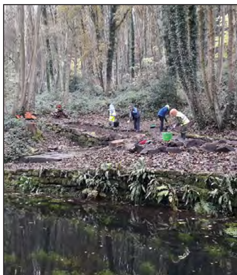
Working on the offside footpath at Robin Hood.
