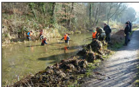
Derbyshire Wildlife Trust volunteers clearing reeds from the offside by dragging them across the canal to the towpath; the bank opposite is too steep to stack them. They were working at "Percy's Cottage" aka Mold's Wharf north of Grattan Bridge, Ambergate.
