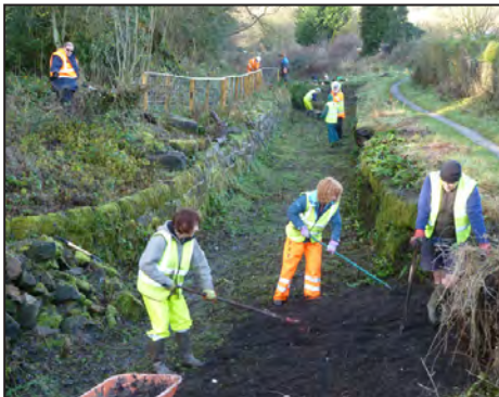
Clearing the gauging narrows at Sawmills. Photo: Hugh Potter
