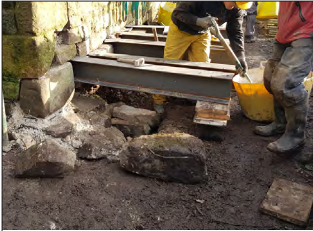
One of the first tasks was underpinning work.
