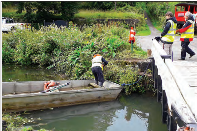
Vegetation clearance at Brown's Bridge at High Peak Junction.
