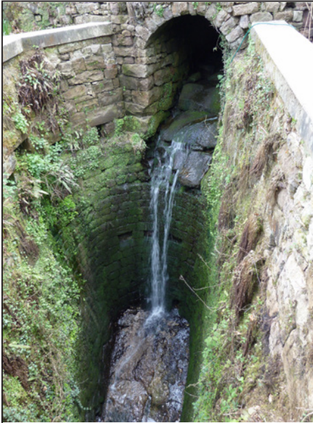
The water of Leashaw Brook still tumbles into the 'bear-pit' where once a turbine was housed to drive the sawmill.
