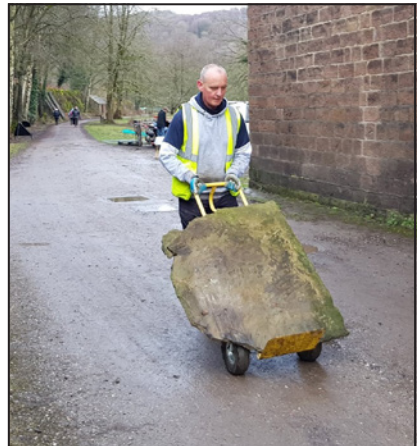
Moving the massive stone roof tiles.
