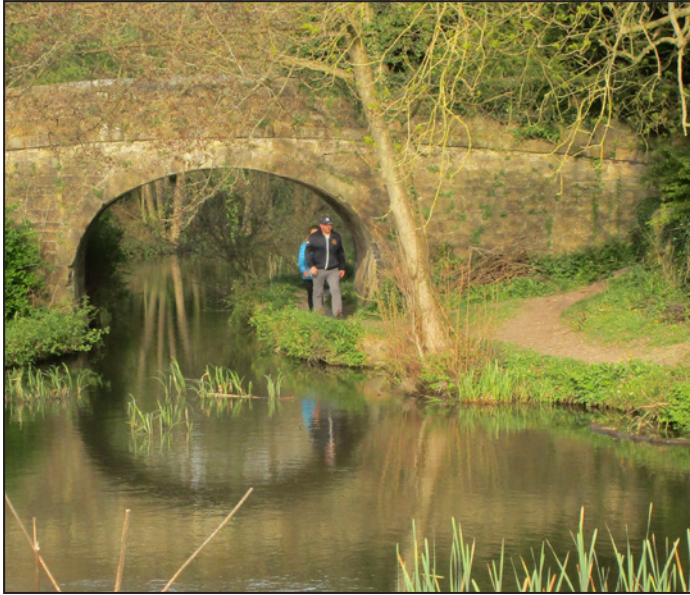
The isolated Starvehimvalley Bridge dates back to the canal's opening in the 1790s.
