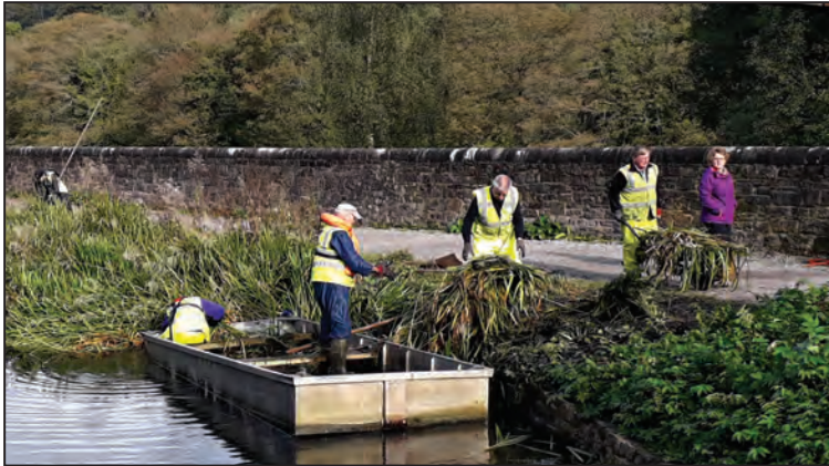
Reed clearance by High Peak Junction swing bridge.
