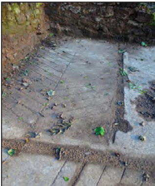
. . . with its distinctive drainage grooves. Photo: Steve Carver
