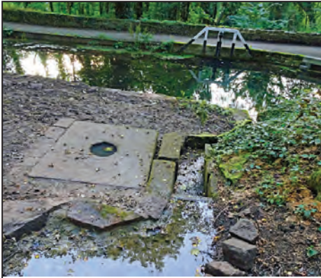
The base of the canalside crane with the small stream to its right which enters the canal by a silt trap. On the towpath opposite is the run-off sluice and adjacent more modern weir.
