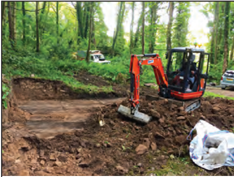
Geoff and his digger reveal the stable floor . . . Photo: Steve Carver
