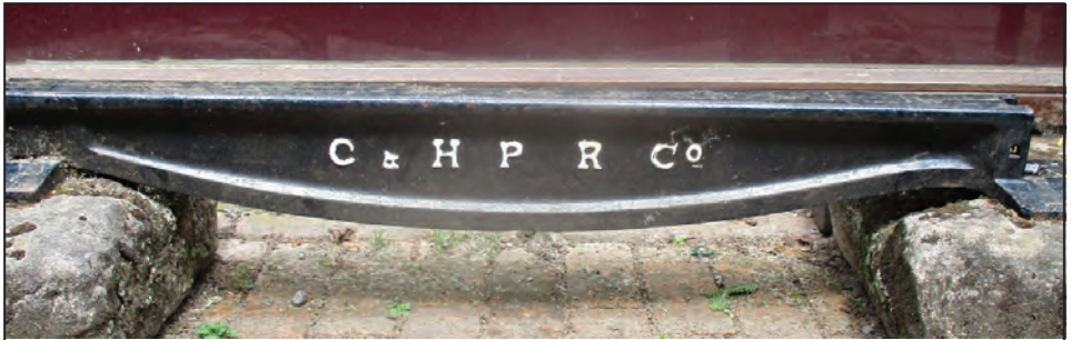
Old cast iron rail seen in the High Peak Junction workshops.
