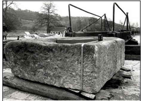
The large pad-stone with the lower ball-race intact.
