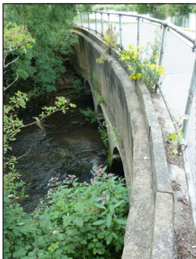
The aqueduct over the River Erewash.
