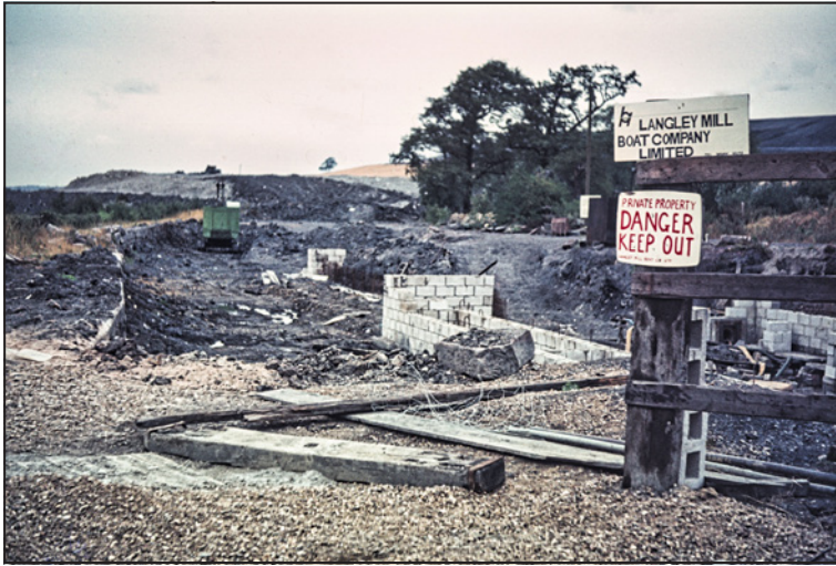
Work was still underway constructing the boatyard above the lock in 1976.
