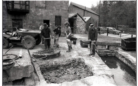
Making foundations for the pad-stone next to the feed.
