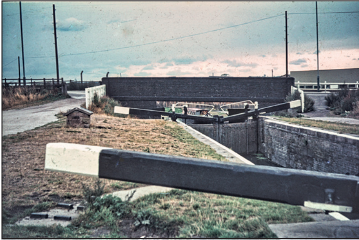
Moored at the head of the Erewash Canal, in fact the very start of the Cromford Canal, below Langley Bridge Lock.
