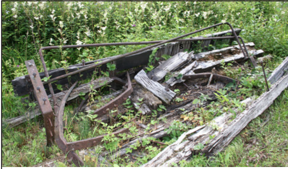
Various bits from the swing bridge and the old icebreaker in a heap on the wharf.
