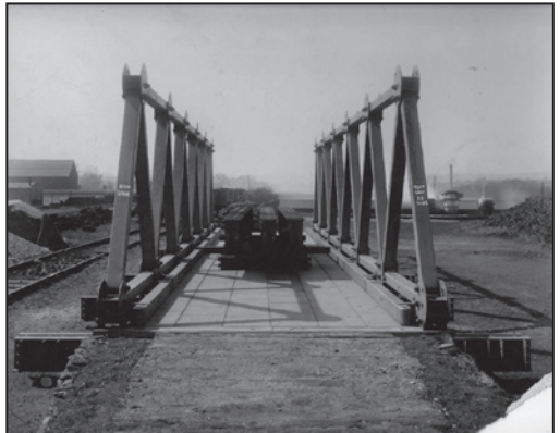
The 60ft span bridge for the Cromford Canal under a 30 ton load test on the Top Plain at Butterley.
