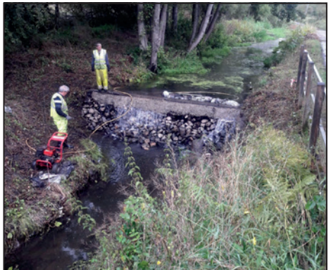
Preparatory work on Pinxton Weir.
