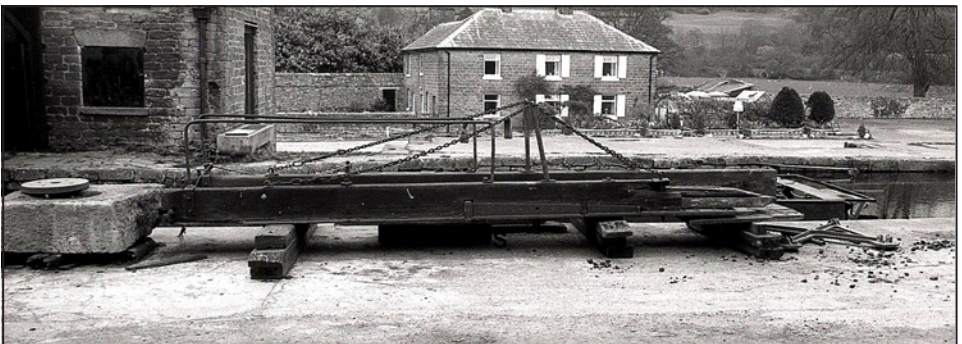
The swing bridge intact alongside the pad-stone at Cromford Wharf.
