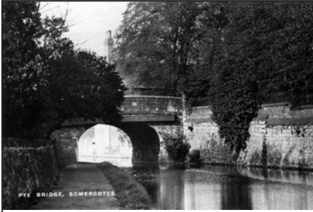
The Alfreton–Nottingham road bridge at Pye Bridge.
