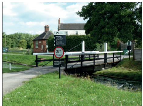
The swing bridge over the Nottingham Canal and toll office at Langley Mill.
