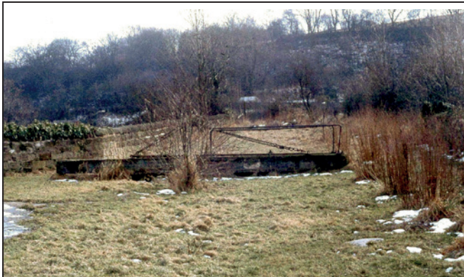
The swing bridge in situ with the aqueduct filled in.
