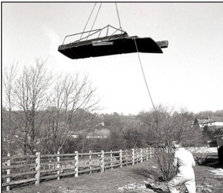
Take off – the swing bridge being lifted away.
