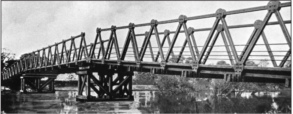
Butterley won the contract for the bridge to Tagg Island on the Thames to give better wartime access to a car factory. Earlier, in 1913, comedian Fred Karnot of Edwardian music hall fame opened his casino on the island (known as the Karsino), which subsequently became very famous, giving stage breaks to many artists including Charlie Chaplin and Stan Laurel of Laurel & Hardy.
