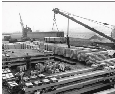
Some of the 400 tons of components for bridges in Angola being loaded on the Top Plain at Butterley.
