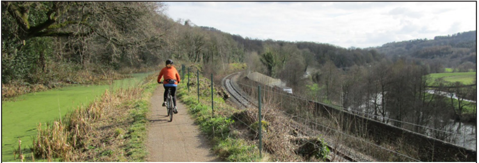
The canal, railway, road and river all vie for space in the narrow Derwent Valley.
