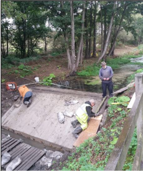
John Baylis supervising work in progress. Photo: John Guyler
