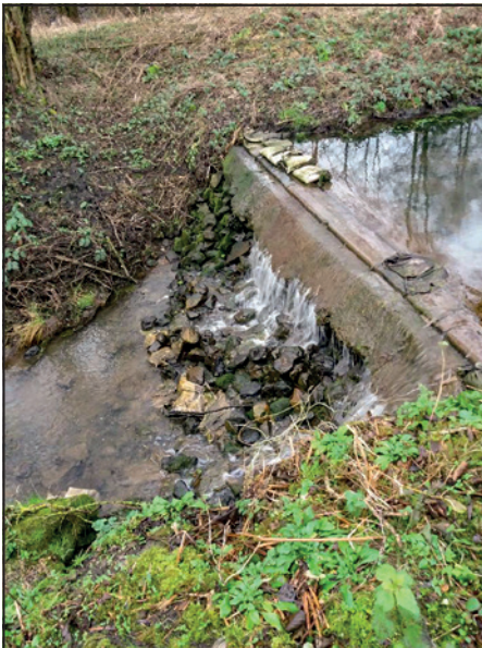
The state of the weir before work began. Photo: John Barker
