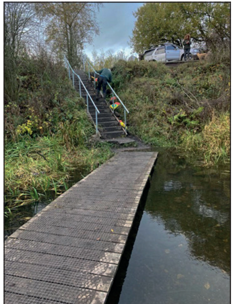
Friends of the Forge fitting handrails to the steps installed by FCC earlier this year.
