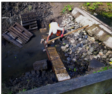
Laying out the slope for the concrete apron. Photo: John Guyler
