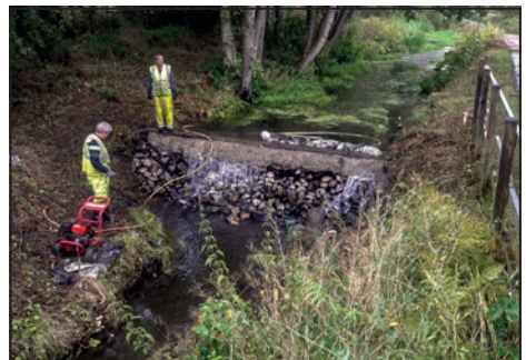
Work begins on Pinxton Weir. Photo: John Guyler
