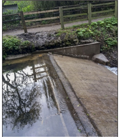
The finished weir. Photo: John Guyler
