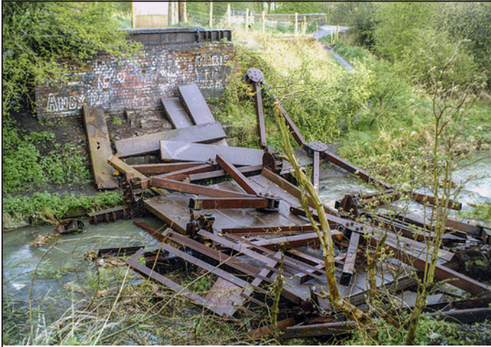
The 'Standard' bridge immediately after demolition.
