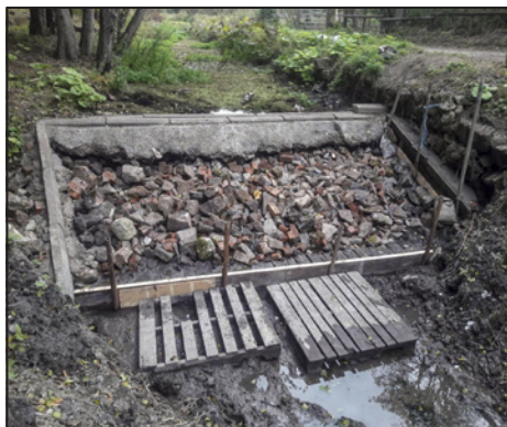
Awaiting the concrete. Photo: John Guyler
