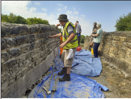
Cleaning up before applying the new mortar. Photo: CRT
