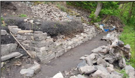
The south garden dry stone wall during reconstruction.
