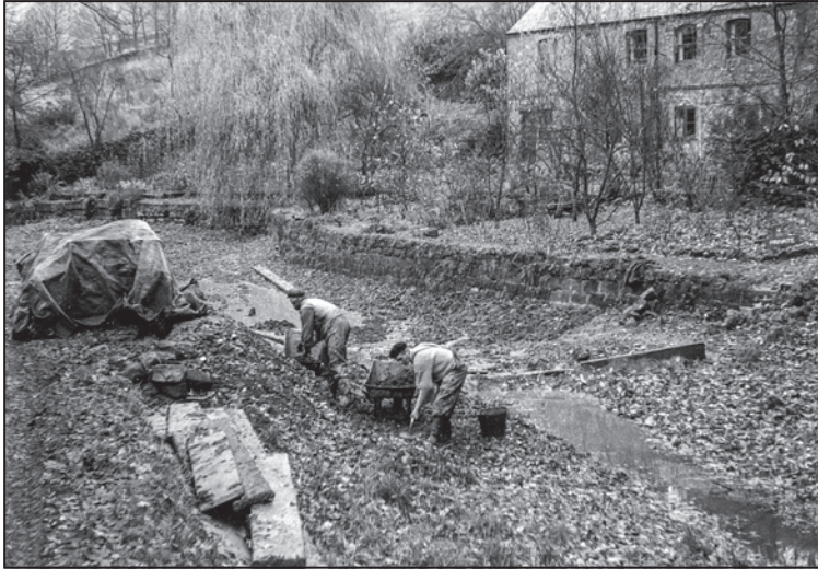
Work to repair a leak at Robin Hood in the 1940s.
