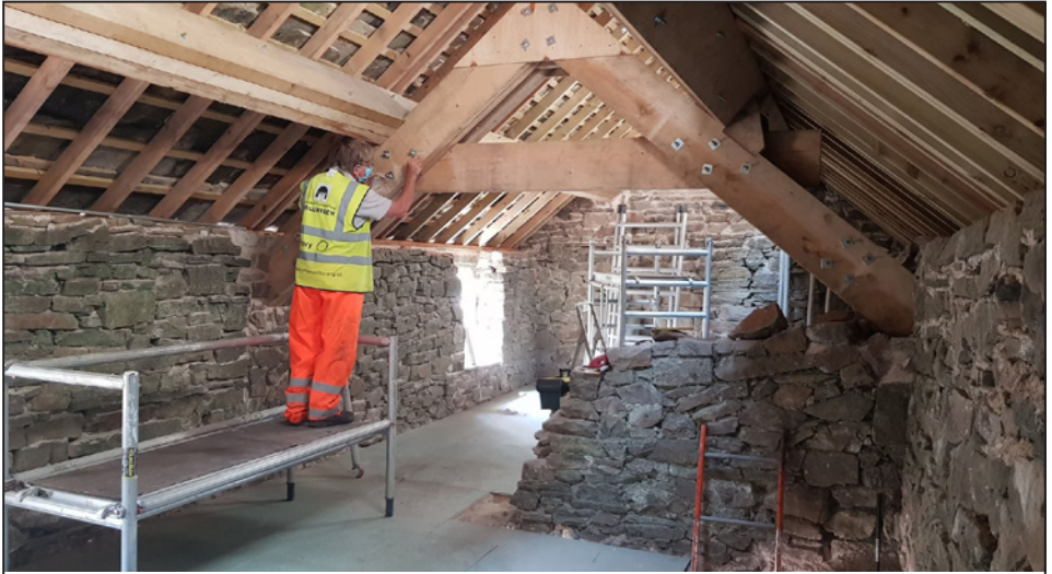
The main timbers were given a rub down to remove unsightly marks.
