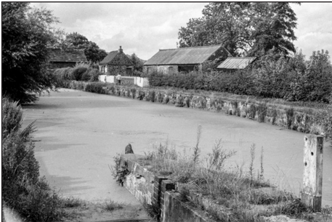
The former canal workshops and the entry to the dry dock by Lock 6, which still retained one of the top ground paddles.
