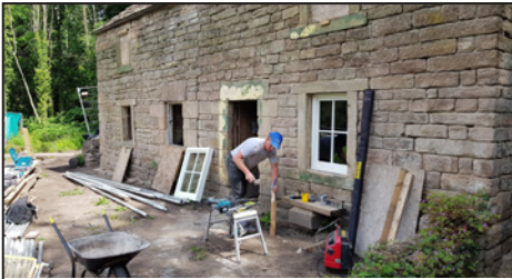
All the units were installed in a single day.
