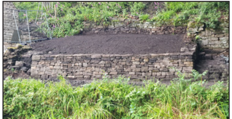
The completed wall. A beautiful new feature in the cottage grounds..
