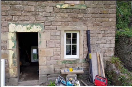
The kitchen window was the first to be installed.
