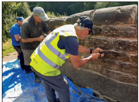
Chiselling out the old mortar.
