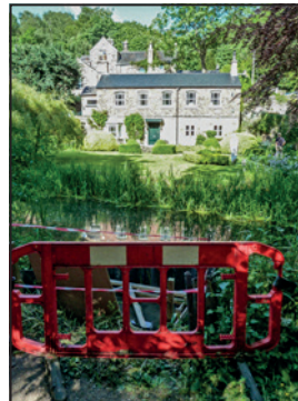
The location of the recent leak, opposite the house, is almost identical to that of the 1940s breach. Note how the garden has changed.
