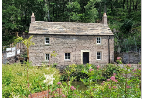
Remember this? Aqueduct Cottage at the start of the project in 2016. These 'before' and 'after' photos had over 120,000 views on the cottage's social media page.
