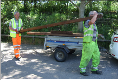
Fence rails being unloaded. Photo: John Guyler
