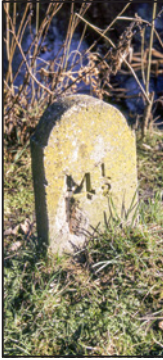
The 4½ concrete post typical of those installed around 1948 photographed in 1997. These were normally placed on the side of the towpath away from the canal where several have survived (including 6 and 10 ½ further down the canal), but this one was placed at the canal edge and recent mechanical mowing has gradually destroyed it so that it is barely discernible today.
