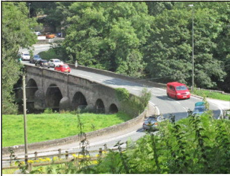
Whatstandwell Bridge; a narrow footway helps keep walkers safe.
