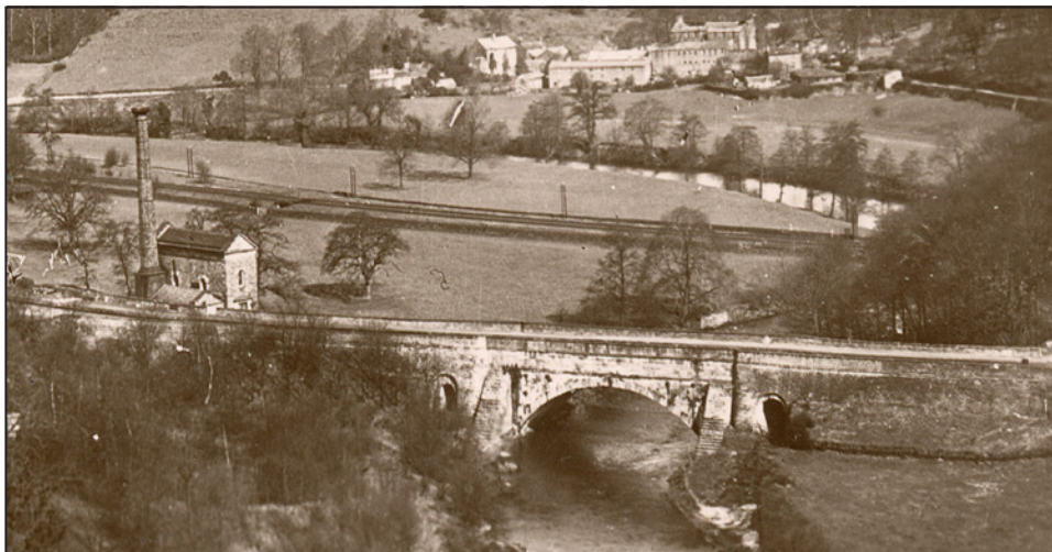
The large buttresses that had to be put in by Jessop to stabilise Derwent Aqueduct can be seen in this high-level view. It was the failure of this aqueduct that delayed the full opening to 1794. Leawood Pump can be seen on the left.
