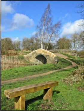
Take a break by 'Humpty Bridge' across the former entrance to Portland Basin.
