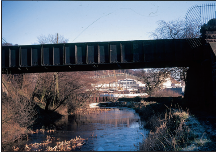
The Ambergate crossing with the canal newly blocked off and the gas works under construction.
