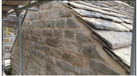
Finished pointing at the apex.
