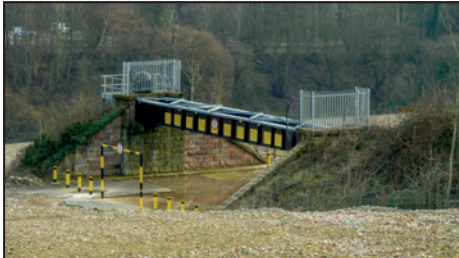
The DVA pipeline bridge across the route of the canal through the former Stevenson's Dye Works site at Bullbridge, currently being developed for housing.
