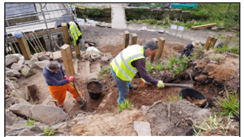
A lot of volunteer hours have gone into rebuilding the stepped path up to Lea Wood
