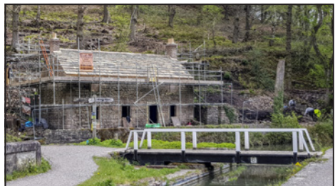
The passers-by view of progress.
