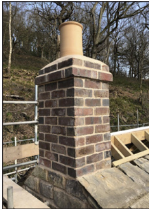
One of the two reconstructed chimneys. Photo: Becky Coleman
