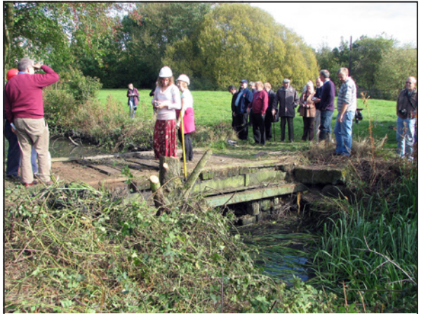
A group from Northern Canals Association examine Palmerston Swing Bridge 13 in 2009.
