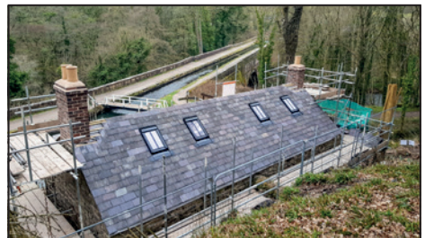
The almost completed slate roof at the rear.
