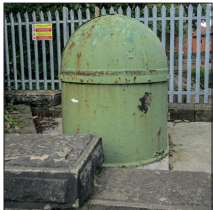
Characteristic green domes track the underground route of the pipeline.
