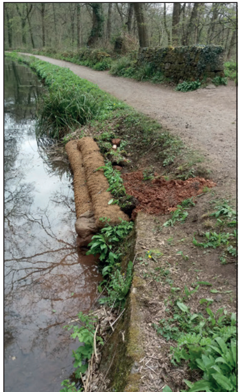
Coir rolls installed to reinforce the bank.
