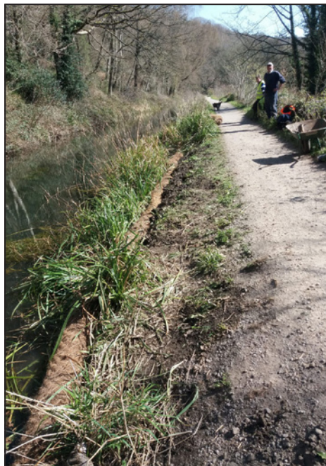
More Coir rolls being fitted near Gregory Tunnel.
