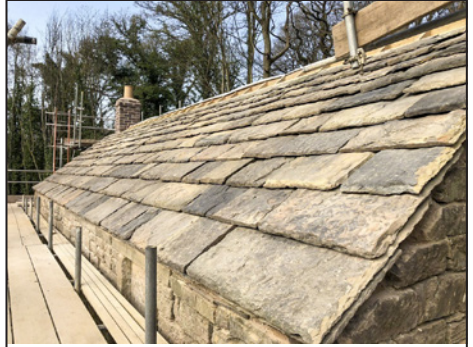
The splendid stone tile roof nears completion.
