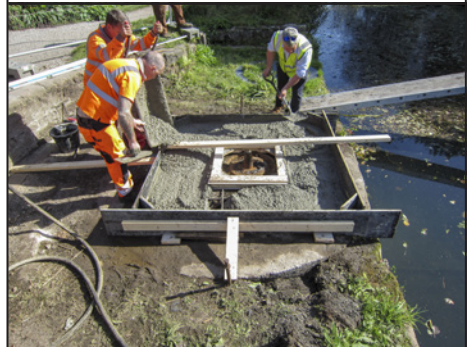
Pouring the concrete for the slewing ring base.
