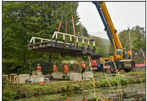
Lifting the bridge for replacement on the slewing ring.
