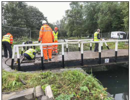
Removing ballast prior to lifting
