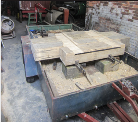
Additional timber required to fit the large diameter of the new slewing ring was obtained from ECPDA stocks at Langley Mill, and cut to shape and preservative treated by FCC.
