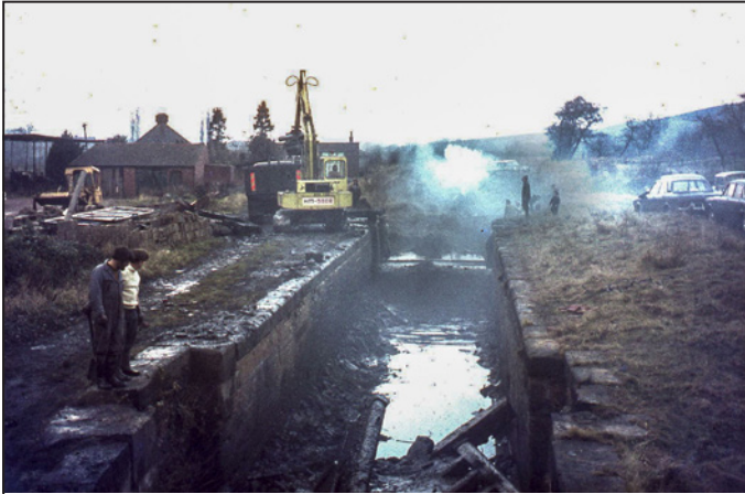
An atmospheric shot of ECPDA's restoration work at Langley Bridge Lock.
