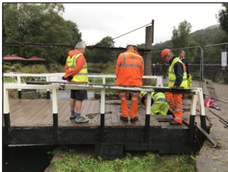
Removing the ballast from Brown's Bridge.
