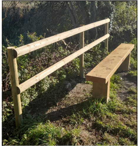
Seat with new fencing to protect the drop to the Hartshay Brook at Hartshay.
