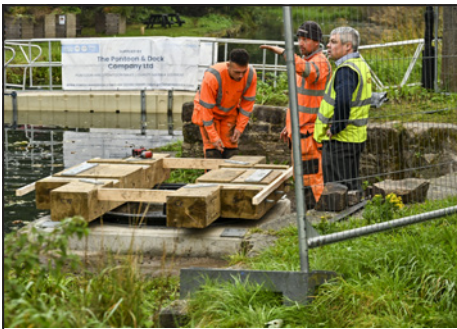
The new timbers being fitted to the slewing ring.
