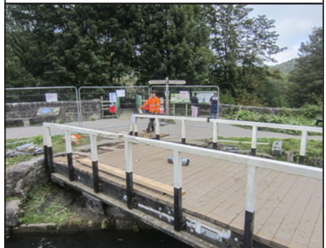
Apprentice Josh demonstrates how easily the bridge can now be swung.
