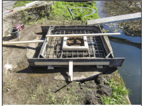
Shuttering for the new concrete base for the slewing ring.
