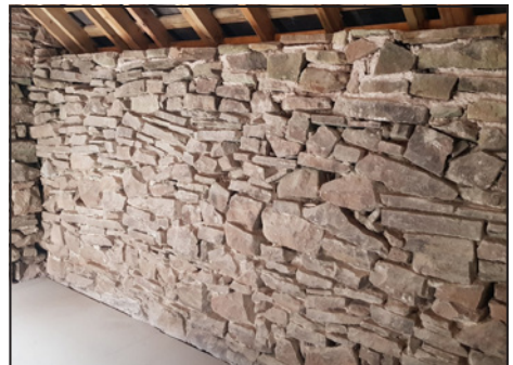
A typical interior wall before lime mortaring.
