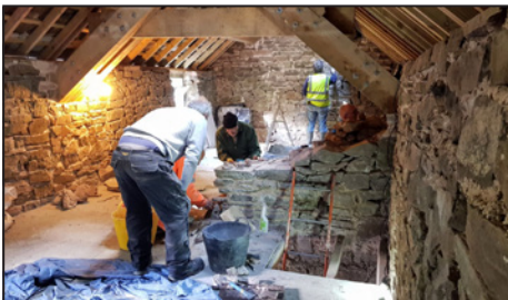
Progress on the upper floor.
