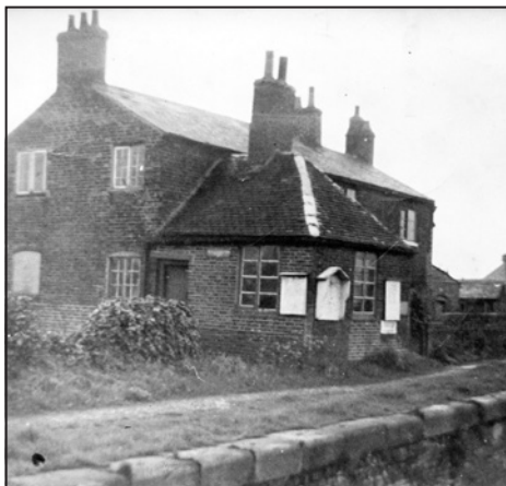
A view from the south showing a second door into the toll office and the extension on the right reduced to one storey. The condition of the cottages here, with noticeboards and lifebelt holder (empty!) is very similar to the one depicted on page 35 of the last issue of Portal which had been taken in 1966.
