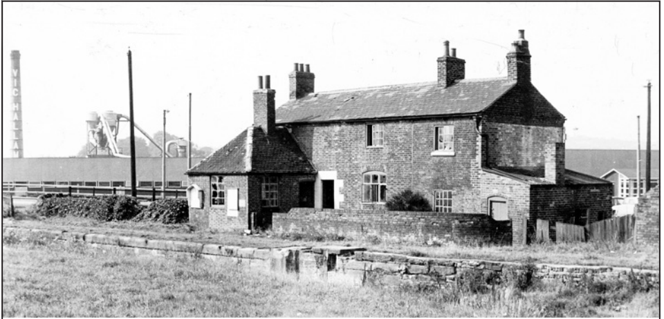
The well-known photograph of the gateless lock with the cottages alongside, shortly before they were demolished. It is clear from this image that the original house had been extended on the right, then a two-storey 'lean to' was added which, by the time of this photograph, had been reduced to single storey.
