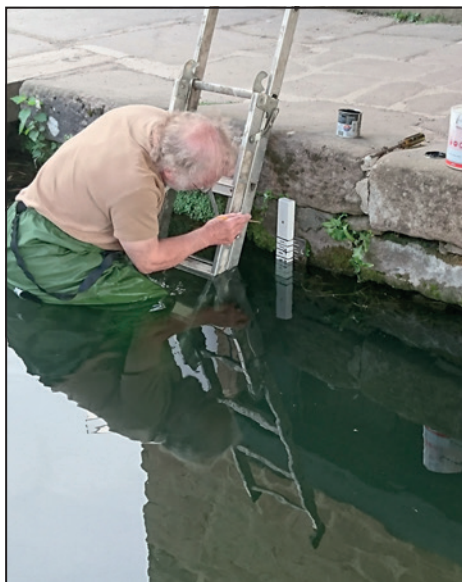
Mike Kelly puts the final touches to the new water level gauge which was installed alongside the earlier less readable gauge.
