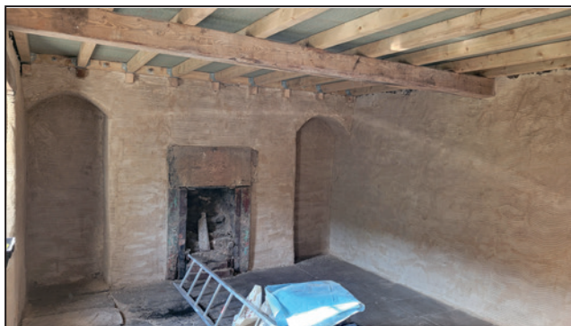
The downstairs room looks bigger after its scratch coat of plaster.
