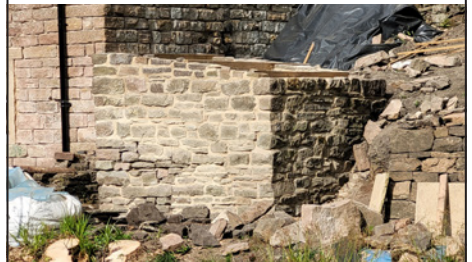
The new lean-to has taken shape.
