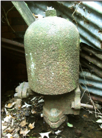
The ram pump that was driven by the water reservoir featured in the last Portal.
