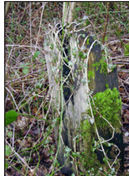
The rotting remains of the windlass that lifted the trap door in the canal bed roughly half-way between Whatstandwell and Ambergate . . .
