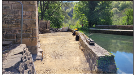
The area at the front of the cottage awaiting flagstones.
