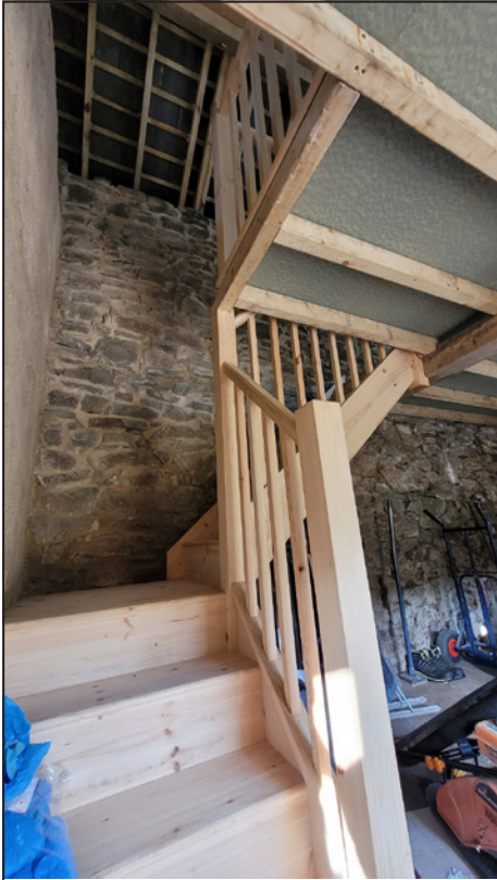
The newly installed stairway to the upper floor.
