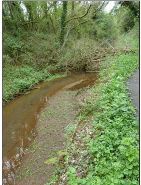
Possibly due to lack of rain in April, the water level in the length to the west of Butterley Tunnel was unusually low.
