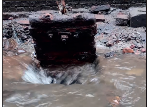
These three stills are from the film The Secret Trap Door Under The Canal showing the dramatic draining of a section of the Rochdale Canal. William Jessop was engineer to both waterways and features such as these and the locks bear many similarities.
