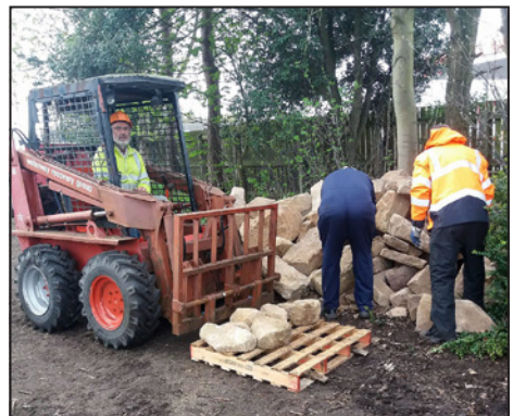
Moving the donated stone at Langley Mill.
