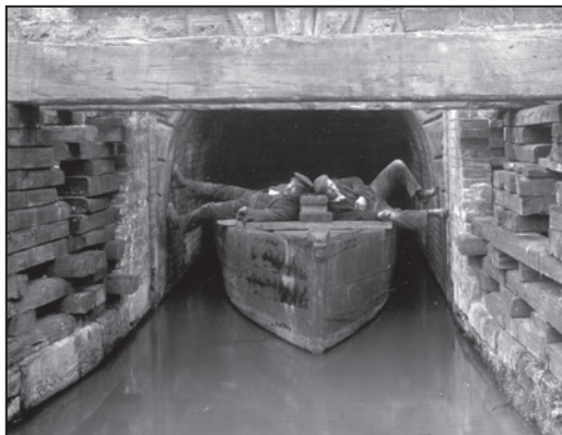
The well-known posed image of leggers emerging from Butterley Tunnel's west end, which is used in the FCC's logo. The photograph dates from 1907, and it is not known if the beams overhead were present in 1862 and so could have been the ones that caused the second fatality.
