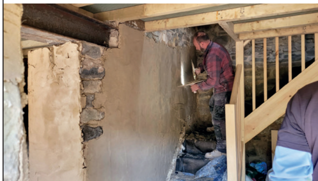
Plastering the stairway.
