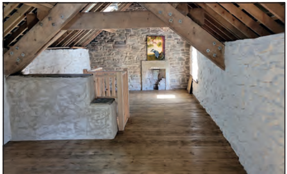
The activity room with floor laid.
