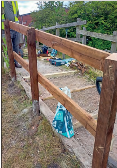
New rails for steps for CRT at Butterley Reservoir.
