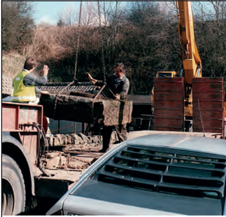
The pivot stone being guided onto the low loader.
