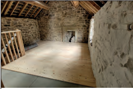
The activity room with access from the new staircase.
