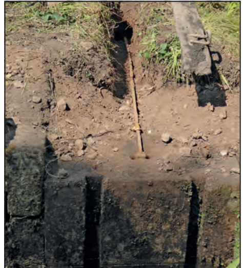
Looking across the canal to the stop plank grooves and the excavated bar.
