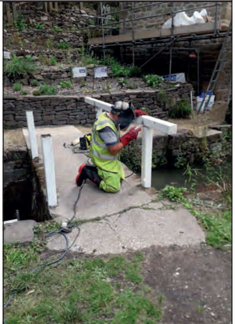
Handrails installed by FCC work party.
