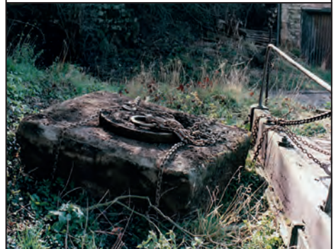
The heavy pivot stone awaiting craning onto the low loader.
