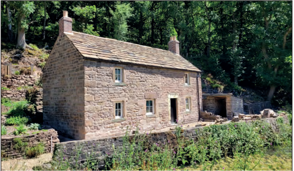
Exterior pointing has transformed the cottage's appearance.
