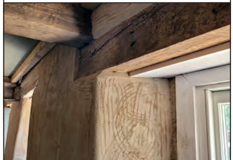
Plastering the interior.
