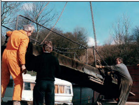
Positioning the swing bridge onto the low loader.
