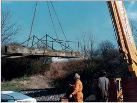
Swinging the swing bridge onto the low loader.
