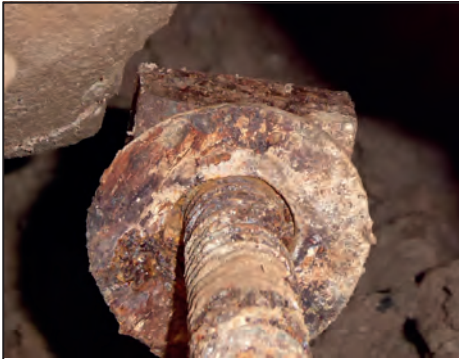
The large nut and washer at the end of the bar.
