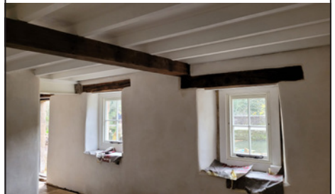
Applying the first of seven(!) coats of intumescent paint to the ceiling.
