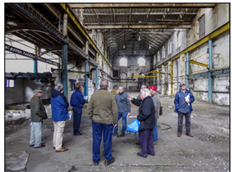
In the massive machine shop, the older part of the building beyond the blue columns is planned to become a heritage centre as part of the site's redevelopment.
