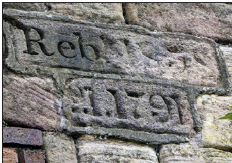
The original date stone of 1791 on one of the furnaces is mounted below one that states 'Rebuilt 1838'.
