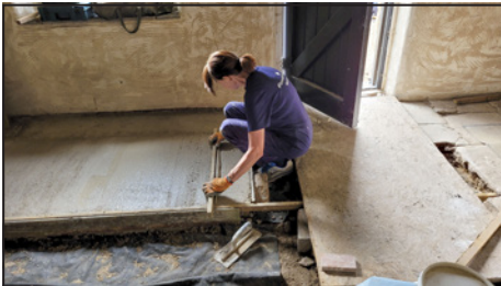
Limecreting the floor.
