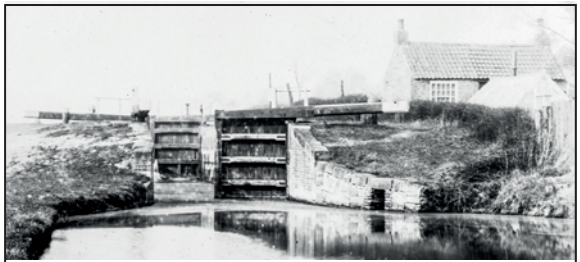
The house and lock (12) by Stoney Lane.
