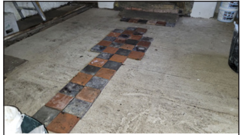
Laying out the tiles on the newly limecreted floor.
