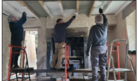
Applying the first of seven(!) coats of intumescent paint to the ceiling.
