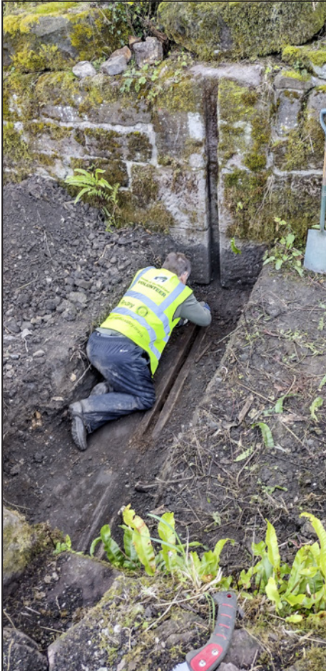
Excavating the base of the stop plank grooves.
