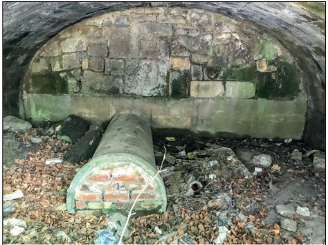
A rare view of the underside of the original Brickyard Bridge.
