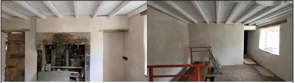
Three coats of lime plaster make a great improvement to the appearance.
