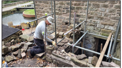
Work starts on the lean-to pantry.
