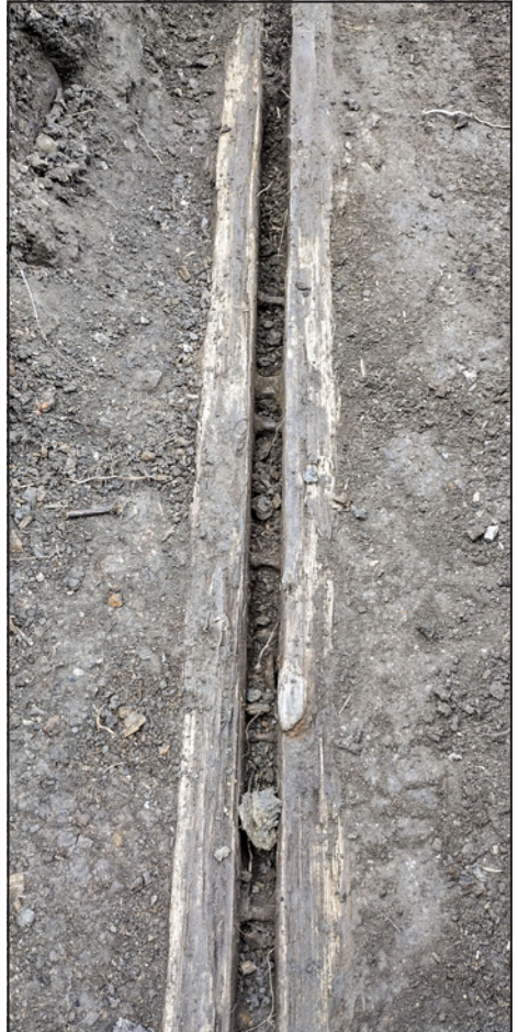
The excavated stop plank base.
