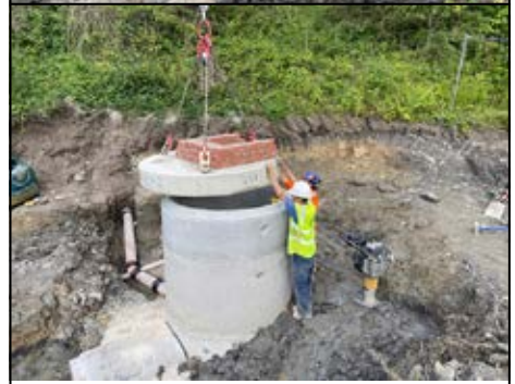
Building the inspection chamber.
