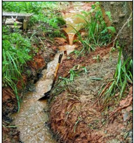
Some of the work clearing the gullies at Moorgreen Reservoir.
