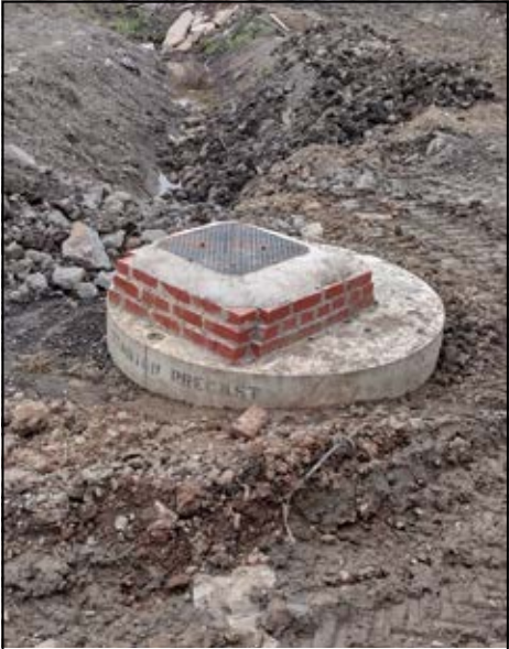
The inspection chamber finished and the surrounding area partially filled in.
