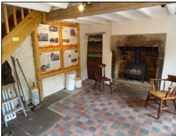
The tiled floor is re-laid and the wood-burning stove installed.
