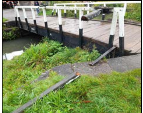
The broken bridge arm.
