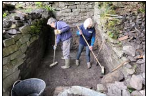
Gradually revealing the old smithy building.
