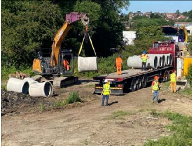
Unloading the concrete pipes.
