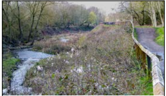
The rise in the towpath marks the site of the top lock at Ironville.
