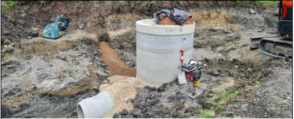
The concrete manhole in place and backfilling is underway.
