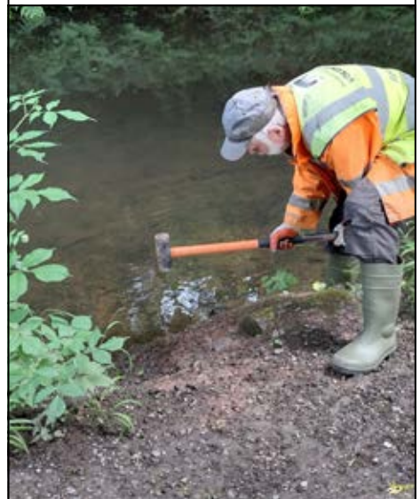
John Dyson hammering a steel pin further in to the coir roll.
