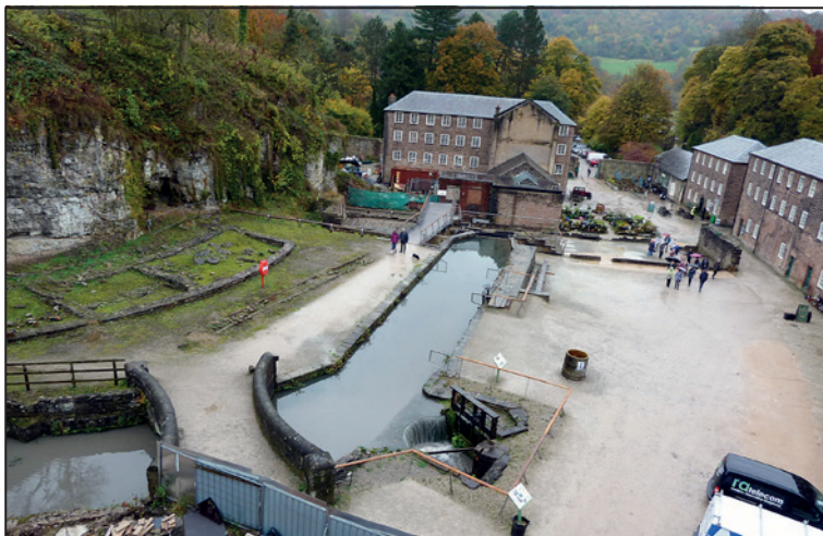
A view from what is now the Cromford Creative building during final work in 2015. The water of the Bonsall Brook, having passed beneath the first mill, flows under the bridge and along the channel to the site of the second wheel pit. On the right of the bridge is the semi-circular weir which takes excess water either to the Derwent or the canal, as controlled by the shuttles referred to in the report.
