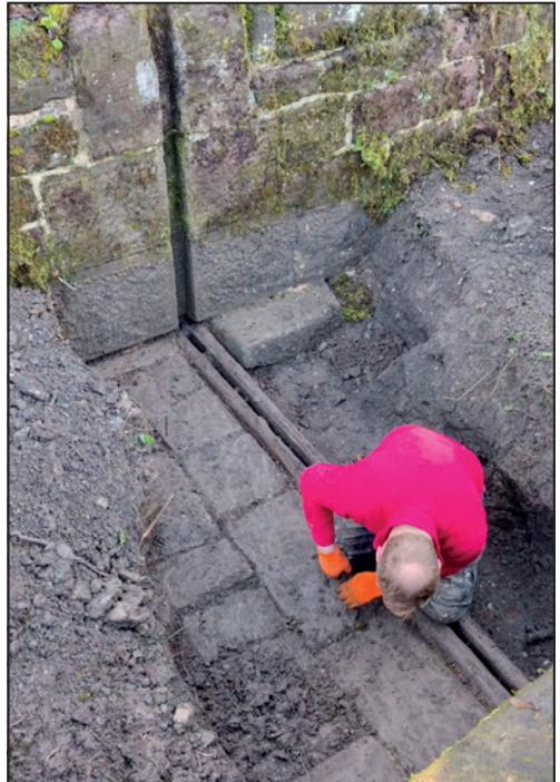
A final clean-up of the stop grooves in the gauging narrows.
