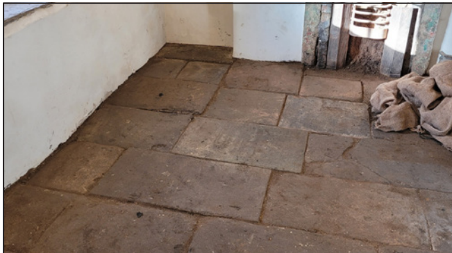
Donated reclaimed flag stones complete the repair of the parlour floor.
