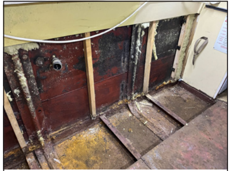
The exposed braces in the galley.
