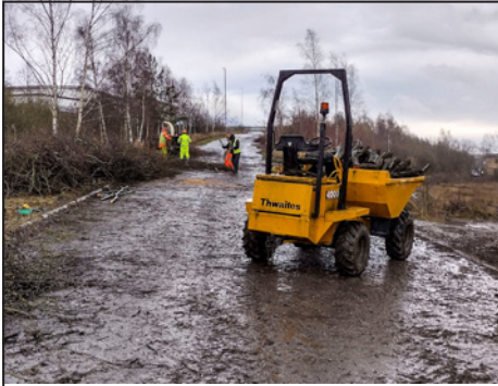
Dumper and chipper at work on Hall Road.
