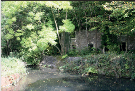
The cottage in 2018 after years of neglect.
