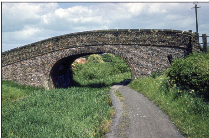
"Bridge 11 carries a rough road to cottages" – seen here a few years after Mr King's visit.
