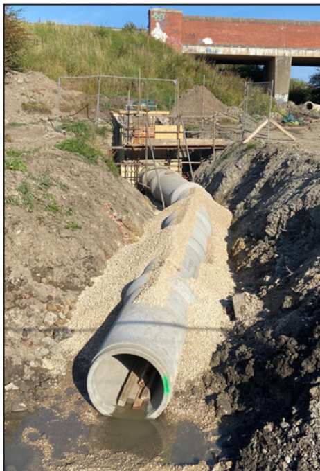
The 900mm pipe trench being filled in.
