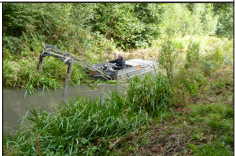
Slowly cutting through the heavy reeds between Ambergate and Whatstandwell.
