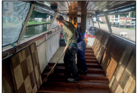
Lifting the floor plates.
