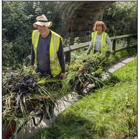
Reed clearance from beneath Ironville Bridge.
