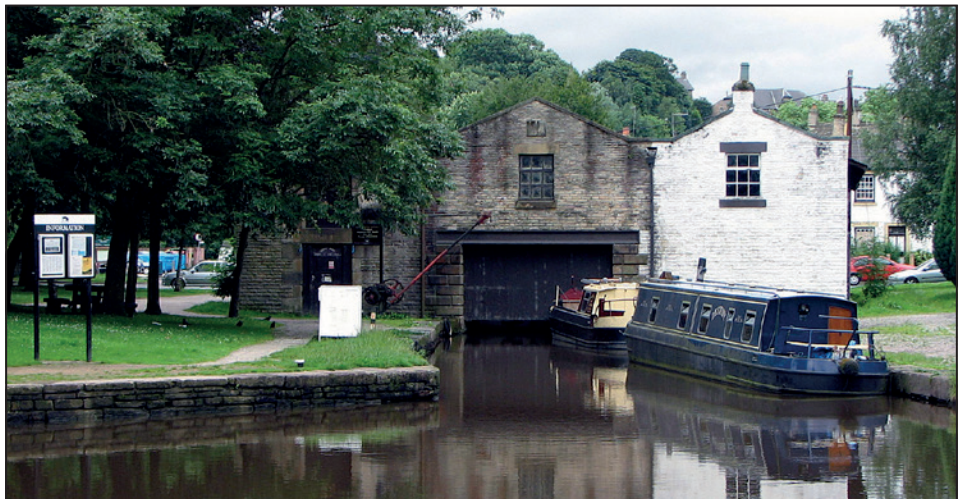
The transhipment warehouse at Whaley Bridge where goods from the CHPR were transferred to/from boats on the Peak Forest Canal, thus enabling a through route for goods between Cromford and Manchester before the main line railways were built.
