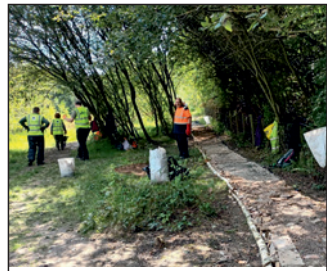
Path building on the Forge site - p8.
