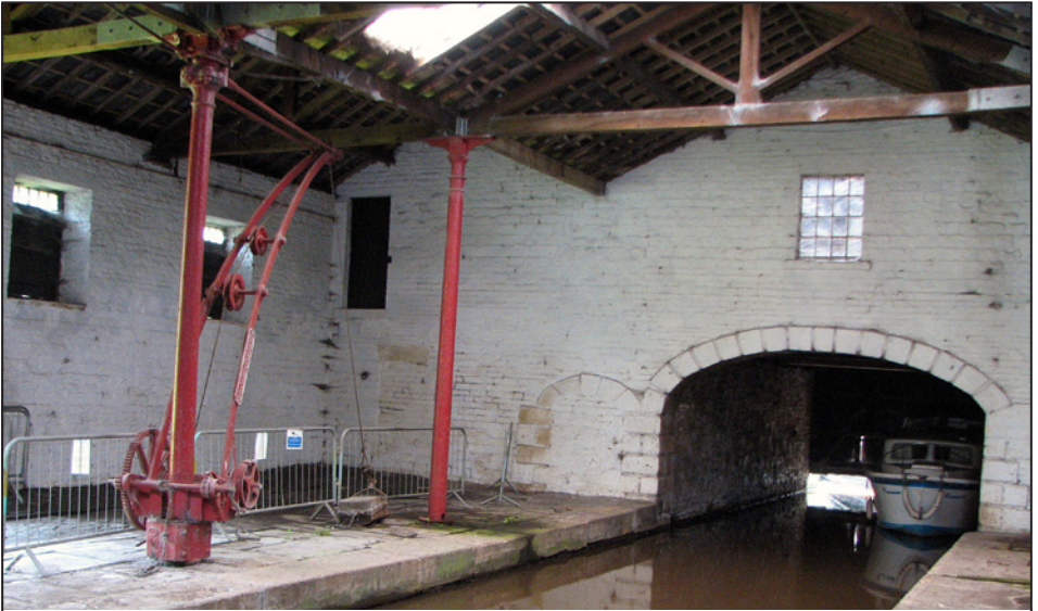
A glimpse inside the transshipment warehouse at Whaley Bridge. On the left is the crane to lift goods between boats and rail wagons.
