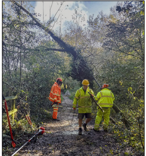
Tree cutting at Codnor Park Reservoir.
