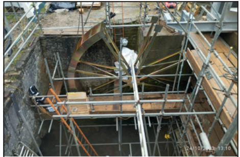
Installing the 5m waterwheel at the end of October.
