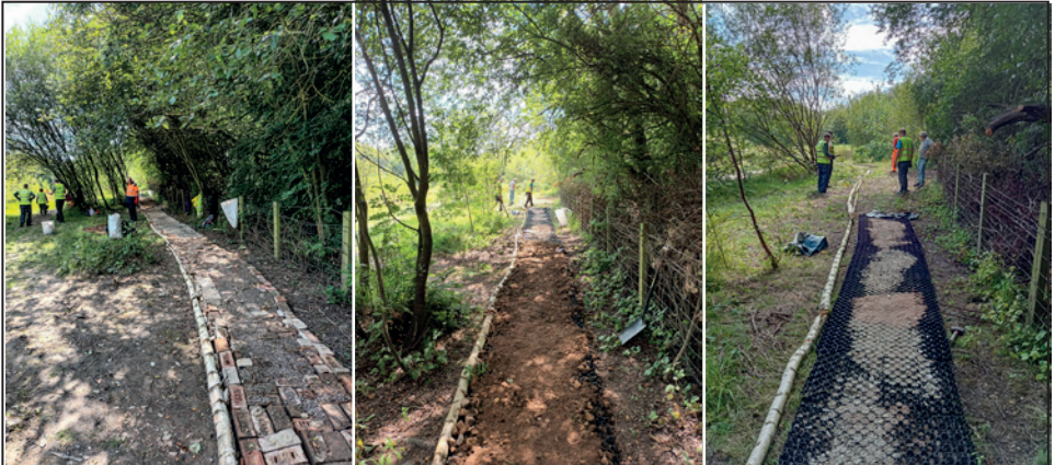
Laying the dry path at the Forge site.
