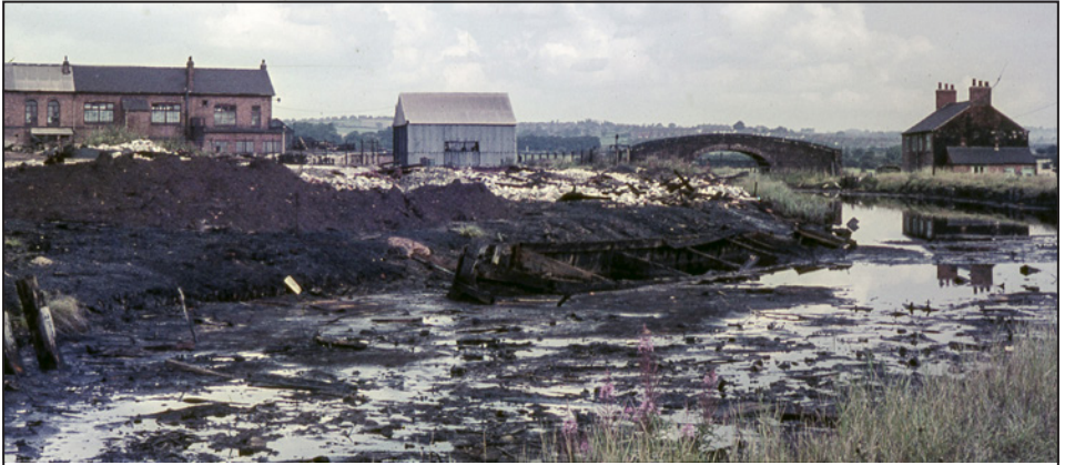
This image sums up the dire description given by Mr King perfectly! Kempson's chemical works is on the left, with Cutts Bridge 10 beyond.
