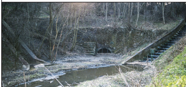
Mr King noted weirs in the form of 'concrete steps' leading into the canal at the eastern entrance to Butterley Tunnel. This 1984 photograph shows the steps on the left, installed in 1907 as a new feed from Butterley Park Reservoir, and those on the right installed in the mid-1930s to take local stream water when the reservoir was drained. Note how silted up the canal is at the tunnel portal.
