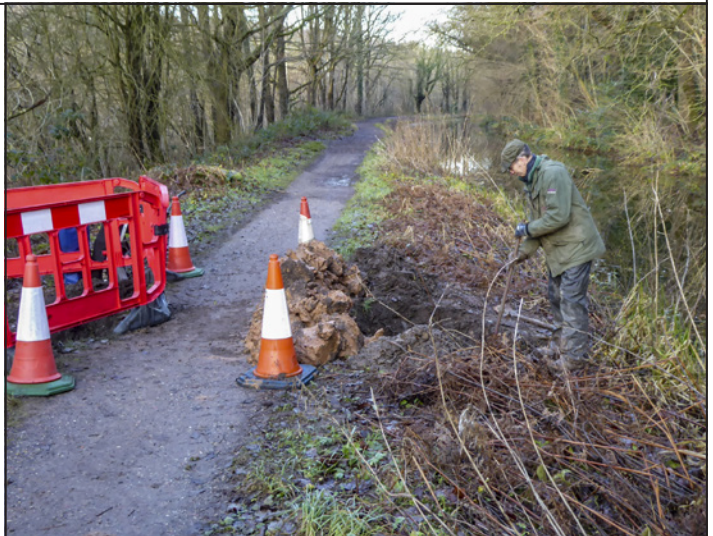
Fixing the leak near Ambergate in January.
