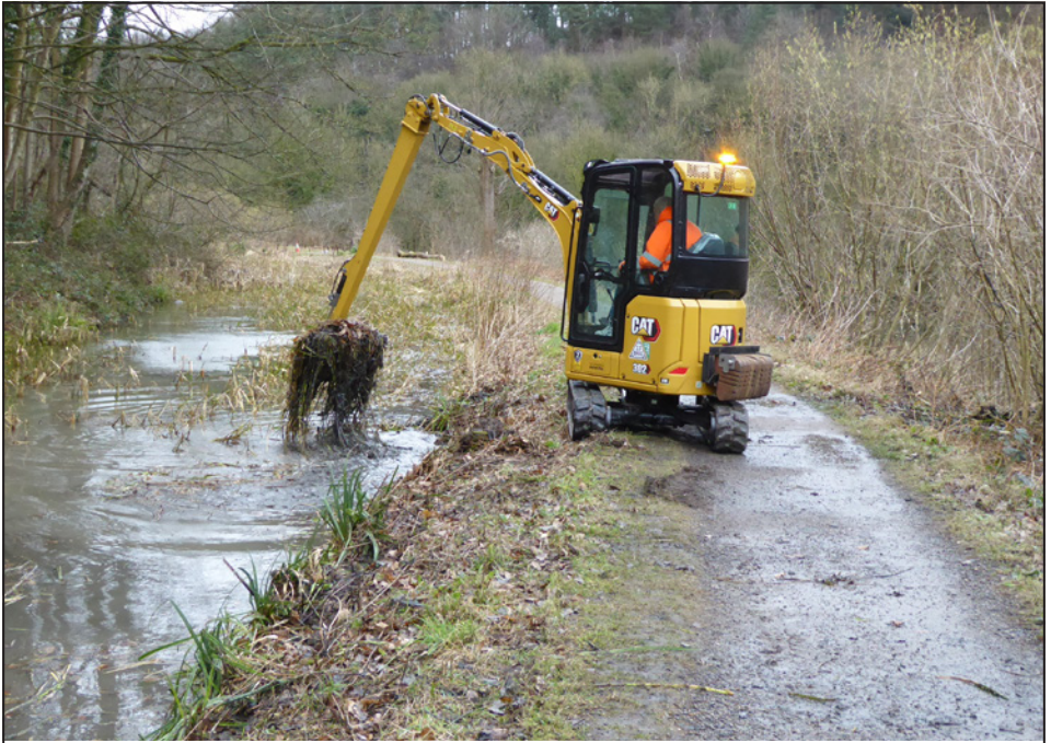
Dredging just south of Aqueduct Cottage.
