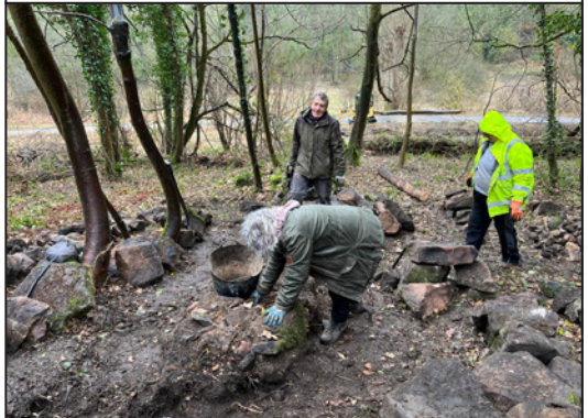
Working on the Top Garden's dry-stone wall.
