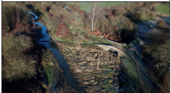
A drone view of Portland Basin Junction and 'Humpy' bridge.
