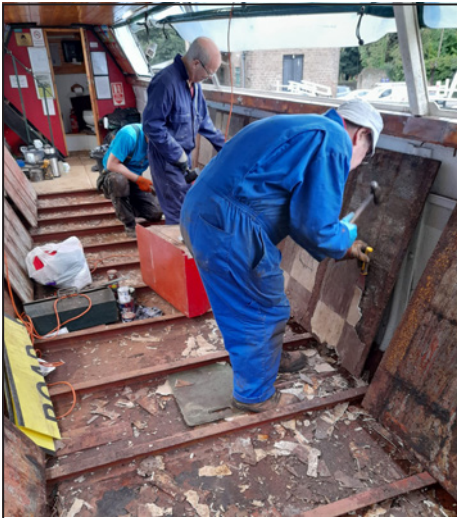
Dave and Norman scraping the old floor tiles off the underside of the floor plates.
