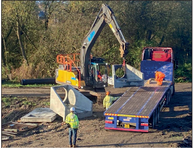
Unloading the headwalls from the lorry at breakfast time!
