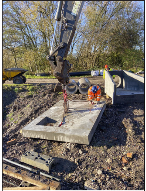
The manhole top plate after unloading.
