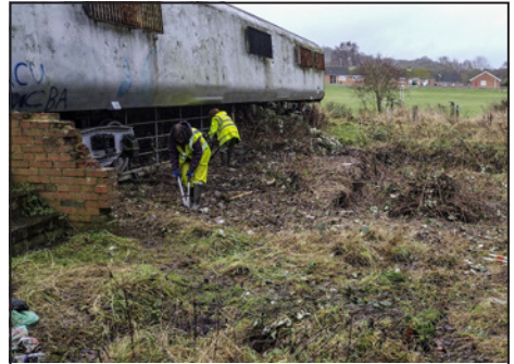
Working on the railway carriage at Ironville.
