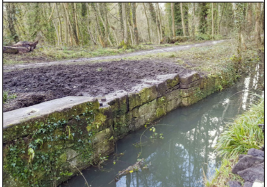
The lock gate recess.
