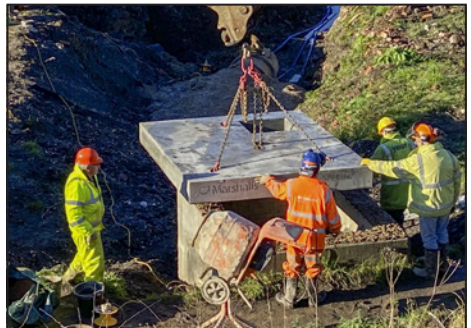
The top plate being lowered into position.
