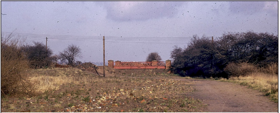
This is the only known photograph of Oakes Tramway Bridge 7 appropriately named as 'Red Bridge' by locals. Curiously it was the adjacent accommodation bridge which was called Red Bridge by the Midland Railway, but which appears to have been demolished by the time this photograph was taken. Do any readers have photographs of these bridges?
