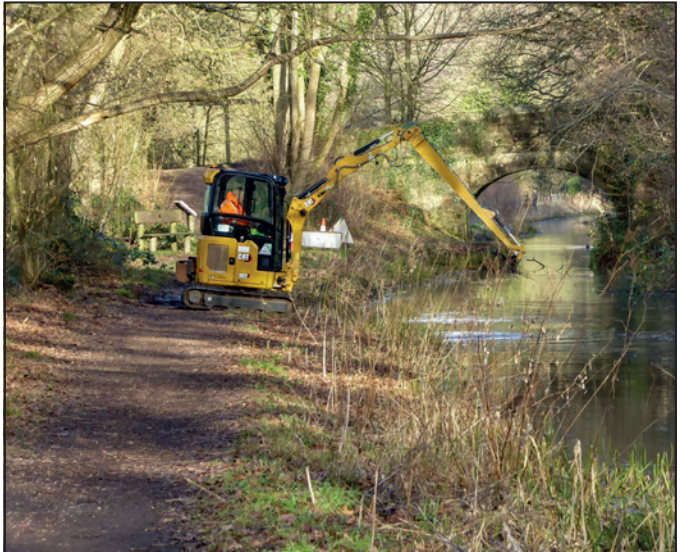
Dredging at Chase Bridge.
