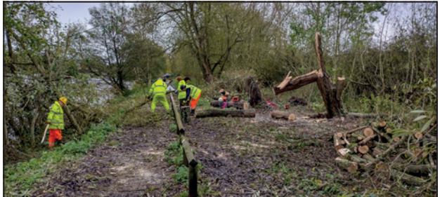
Clearing fallen trees from alongside Codnor Park Reservoir.
