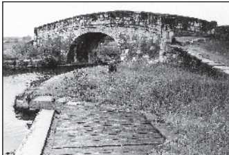
Mr King's inspection covered from Pinxton to Butterley Tunnel - p28.
