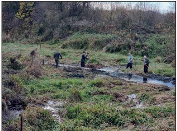
Reed bunding to prevent flooding and path erosion.
