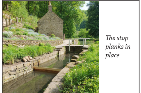
Putting in the stop planks to enable the gate recess to be drained for the fitting of the lock gate.
