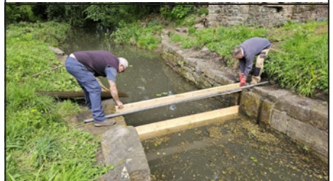
Putting in the stop planks to enable the gate recess to be drained for the fitting of the lock gate.
