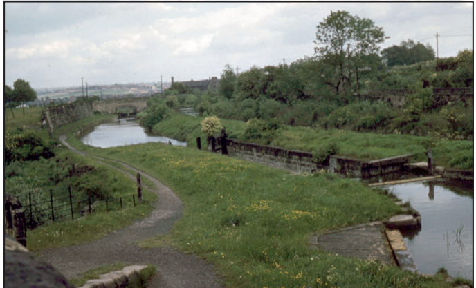
The weir above Top Lock is clearly seen a few years after Mr King's visit, and what remains of the gates are still holding water.
