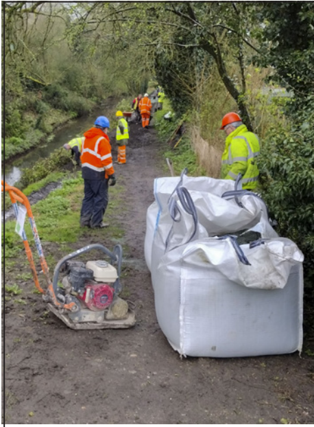
Preparing to lay the granite chips at Hartshay.
