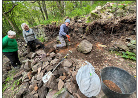
There are plenty of stones to replace in the garden wall.
