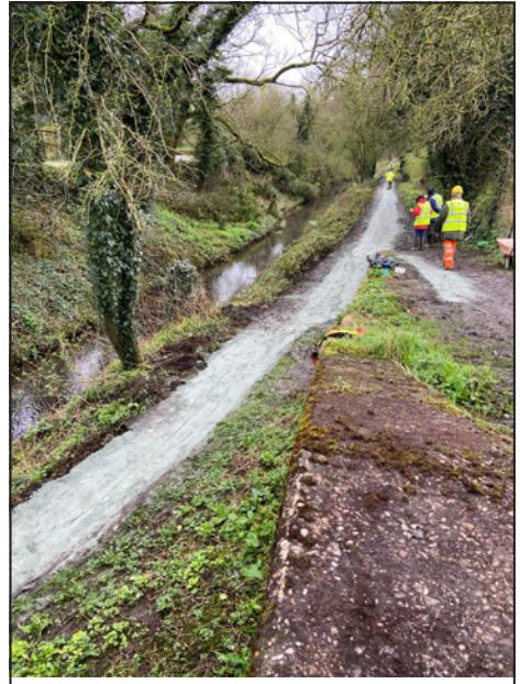
Hartshay towpath after being re-laid.
