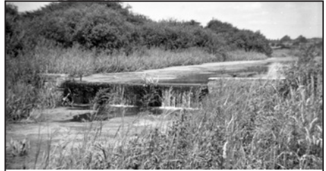
Above Lock 8 Mr King noted this dam with stop boards in the gap. Today that gap is a concrete cill.
