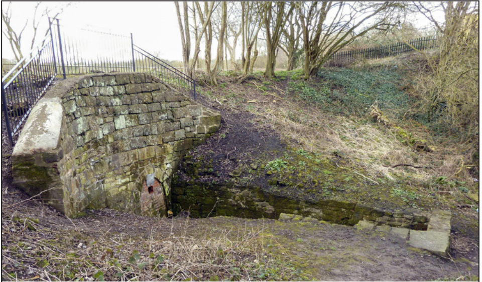
The former outlet sluice channel from Codnor Park Reservoir, which is in the background of this photograph.
