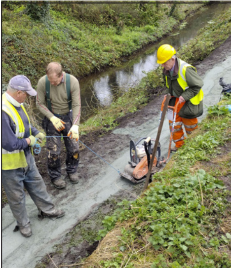
Work to improve the towpath at Lower Hartshay.
