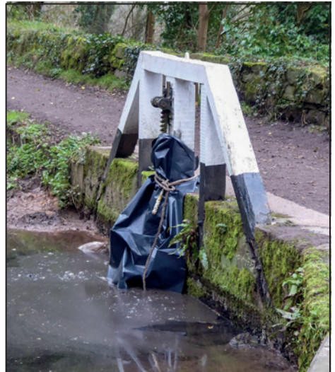
The sluice at Sims Bridge has been replaced.
