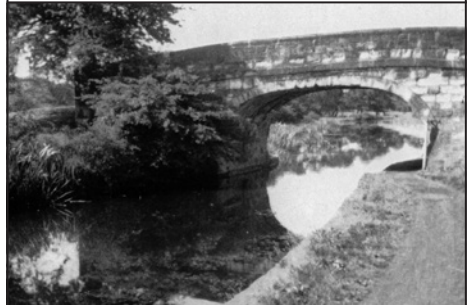
The only known photograph of Slaley's Bridge 40 which was demolished in 1959, despite Mr King's report that it was "in good condition".
