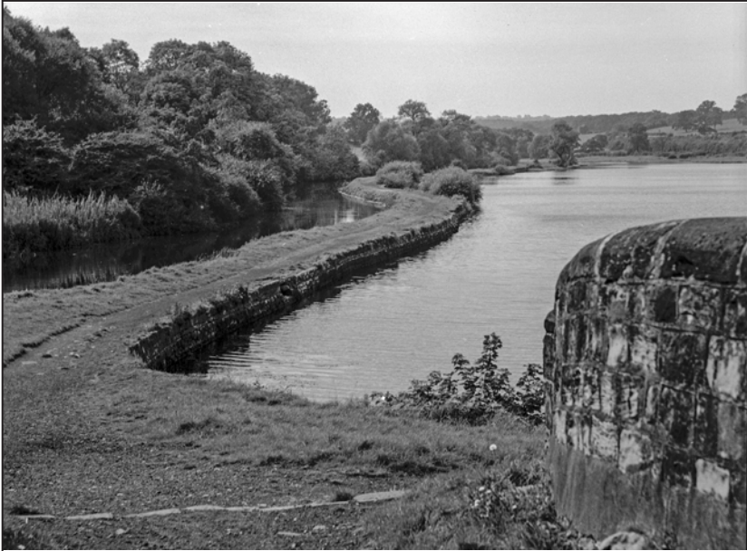
Seen from the Pinxton Arm junction bridge the main canal to the left is separated from Codnor Park Reservoir only by the narrow towpath. In the 1980s the canal was infilled and the reservoir lowered.
